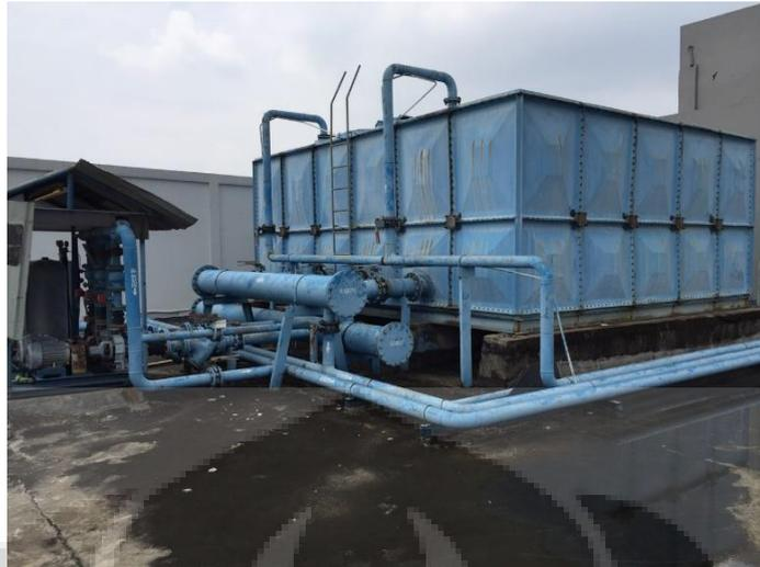
Gambar 4. 6 Tangki Air Atas (*Roof Tank*)
