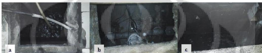
Gambar 3. 3 (a) *sump pit*, (b) *sump pit grease trap*, dan (c) outlet IPAL
