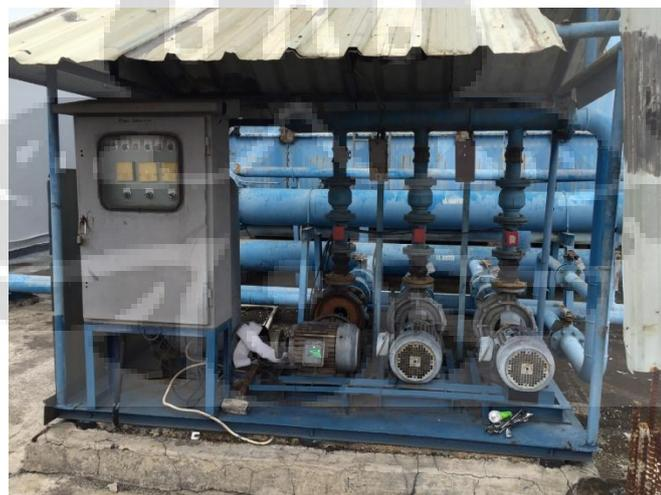
Gambar 4. 7 Pompa Distribusi (*Booster Pump*)
