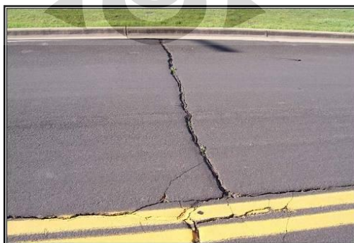
Gambar 2.20. Transverse cracking
