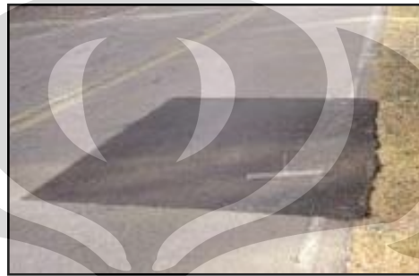
Gambar 2.21. Patching deterioration
