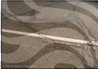
Gambar 2.3. Crack sealing
