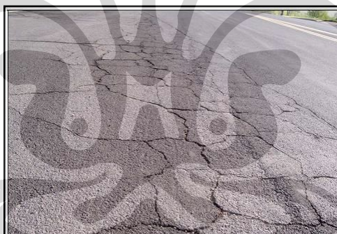
Gambar 2.18. Block cracking
