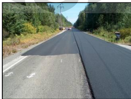
Gambar 2.5. Kegiatan rehabilitasi mayor ( overlay )
