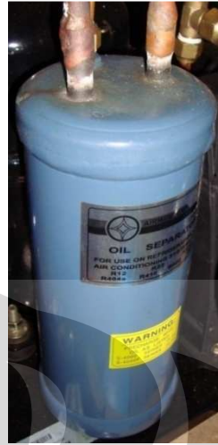
Gambar 3.17. Oil Separator
