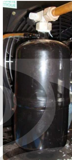
Gambar 3.6. Liquid Receiver
