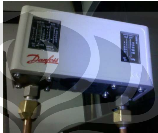
Gambar 3.15. Pressure Control
