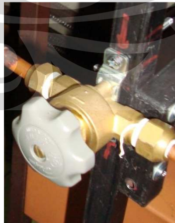
Gambar 3.14. Shut-off Valve
