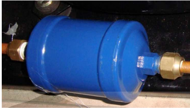
Gambar 3.11. Filter Dryer
