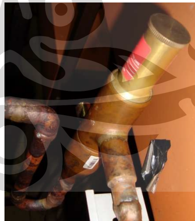
Gambar 3.18. Evaporator Regulator
