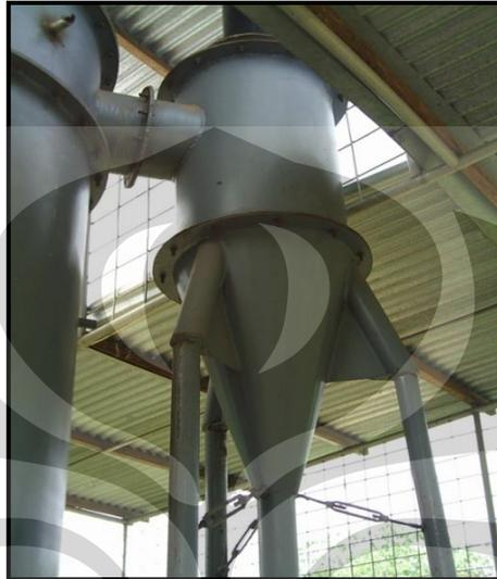
Gambar 2.13 *Cyclone Separator Fluidized Bed Combustor UI*
