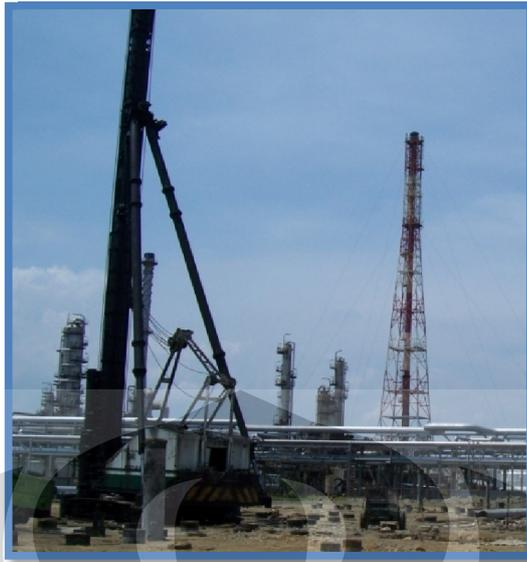
Gambar 2.3. Alat *Pile Rig*
