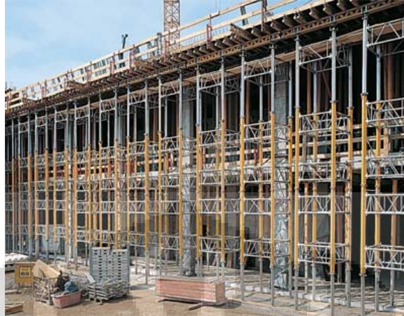
Gambar 2.32: Sistem PERI Multiprop ( www.peri.de )
