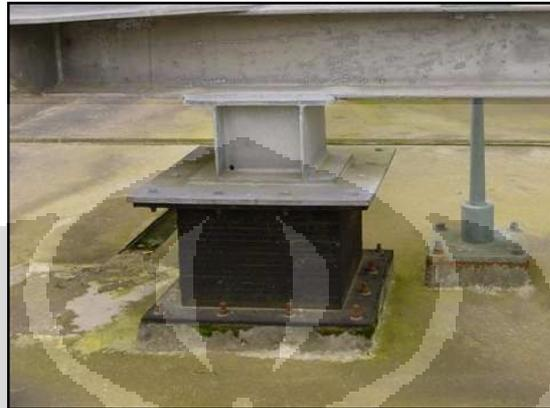
Gambar 2.9. Base Isolator Tipe Elastomeric Bearing
