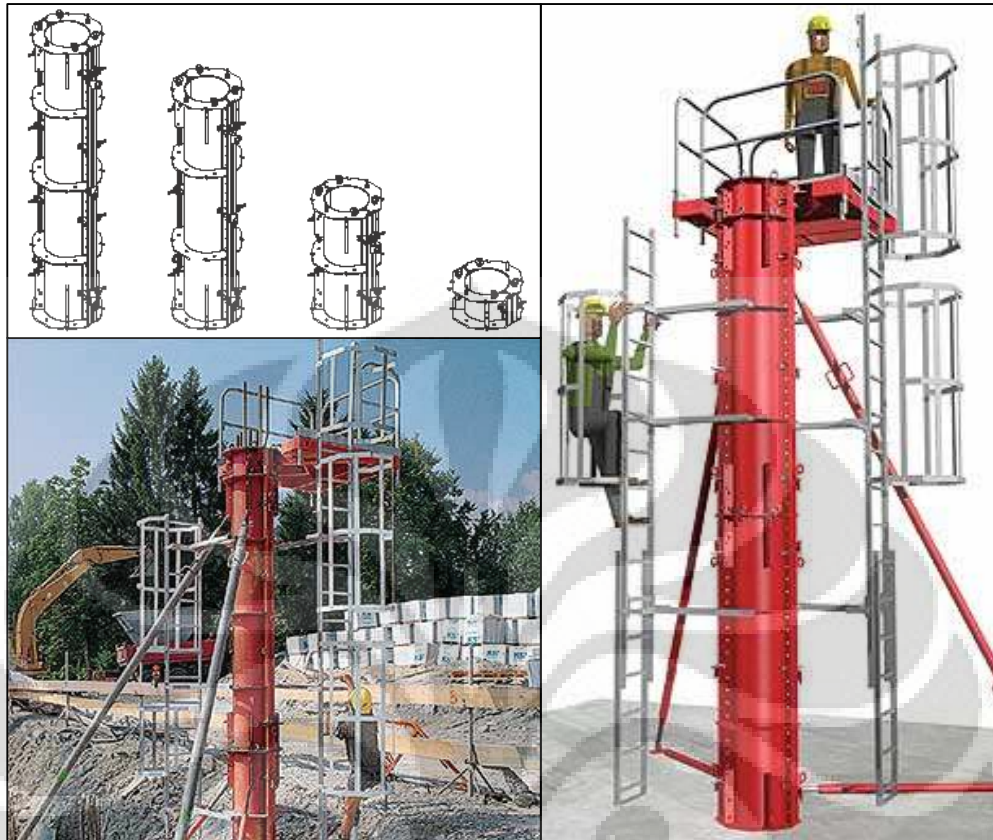
Gambar 5.3 Bekisting Pilon
