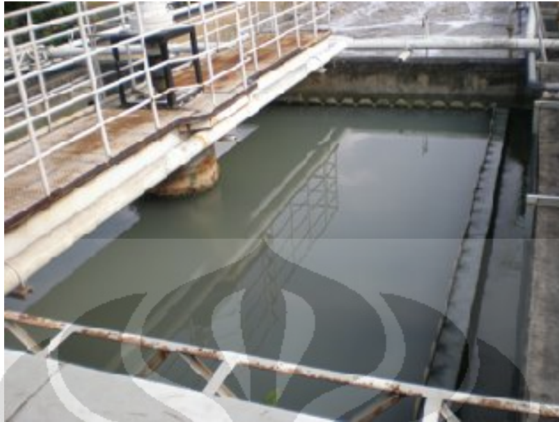
Gambar 4.6. Clarifier Tank
