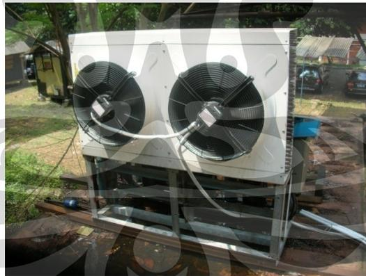
Gambar 2.7 Kondenser *air cooled*
