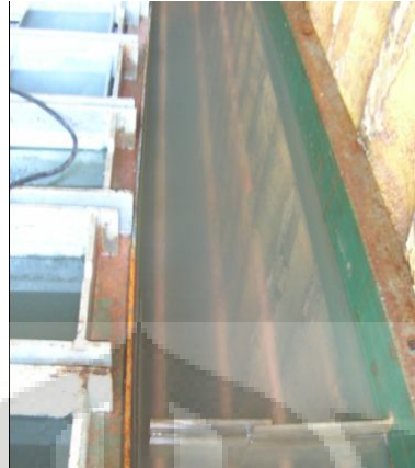
Gambar 3.12 posisi evaporator didalam ice bank
