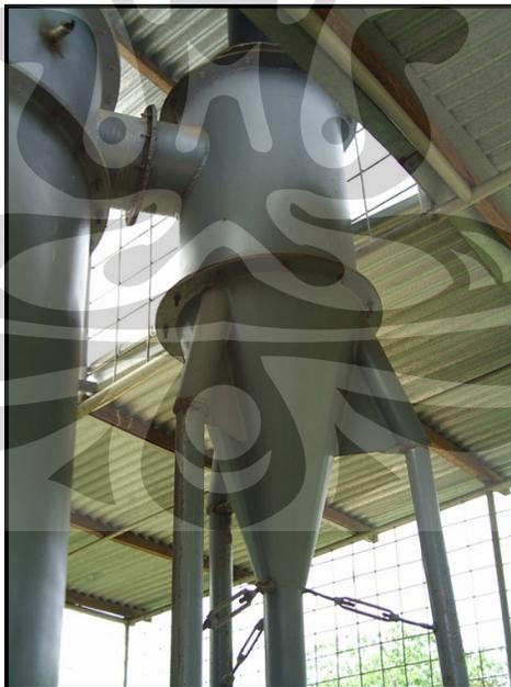
gambar 2. 16 *Cyclone Separator Fluidized Bed Combustor UI*
