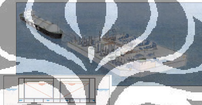
Gambar 2.2 Terminal LNG receiving terminal model Gravity Based Structure
