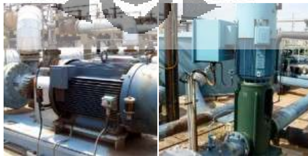
Gambar 2.9 Pompa Sentrifugal (Wikipedia, 2010)
