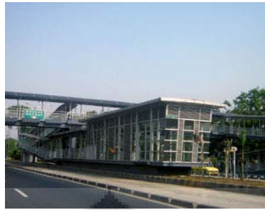
Gambar 3.2 Halte/ Shelter Busway
