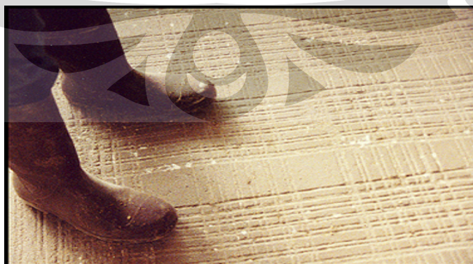
Gambar 2.9 Lantai Beton Beralur
