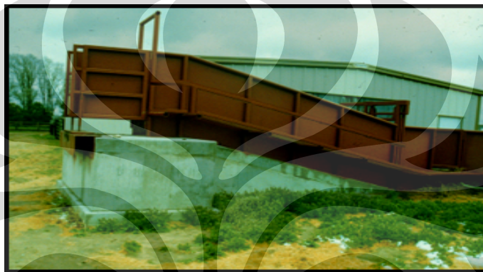
Gambar 2.7 Tampak samping Loading ramp
