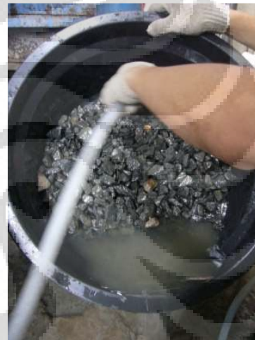
Pencucian Agregat Kasar
