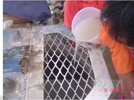
Lampiran B – 2 Gambar proses pengecoran beton geopolimer
