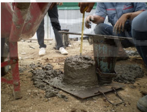
Pengujian slumb beton proyek A (molen 2, slump : 13 cm)
