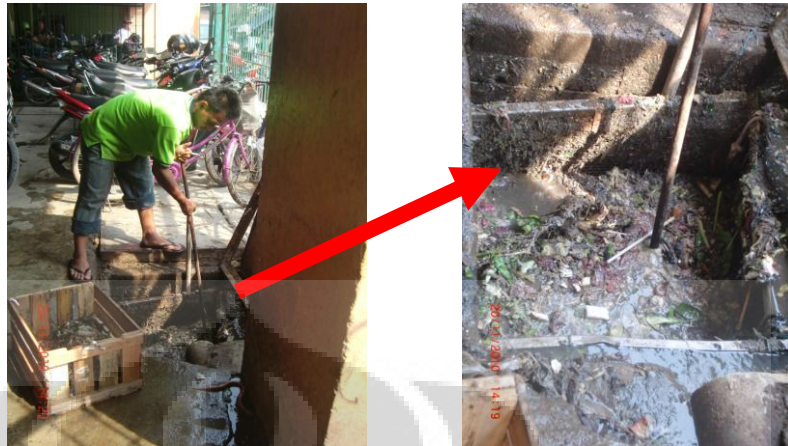
Gambar 4.23 coarse bar screen
