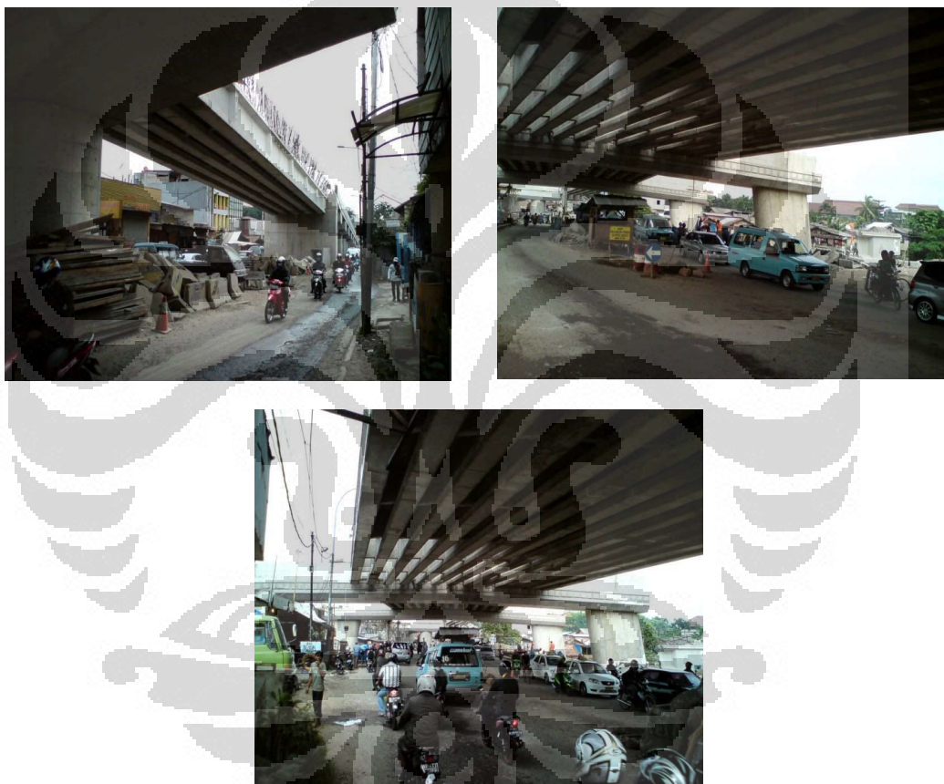
Gambar 3.2 Kondisi Jembatan Flyover Kalibata (8 November 2010)
