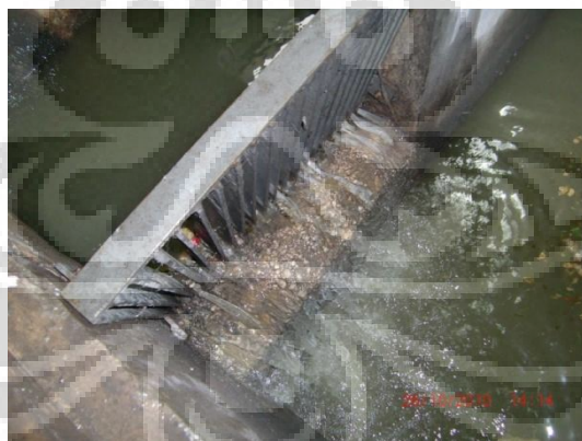
Gambar 4.13 Unit Bar Screen
