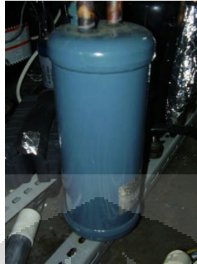
Gambar 3.10 Oil separator
