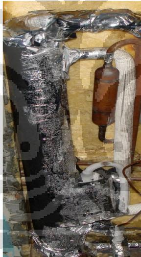
Gambar III-5 cascade heat exchanger
