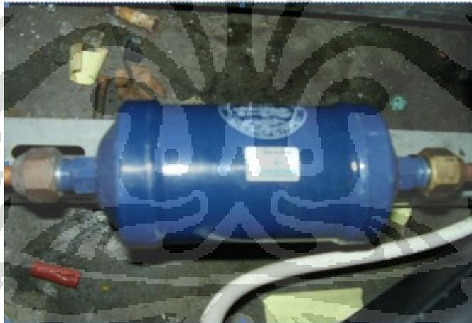
Gambar III-9 filter dryer
