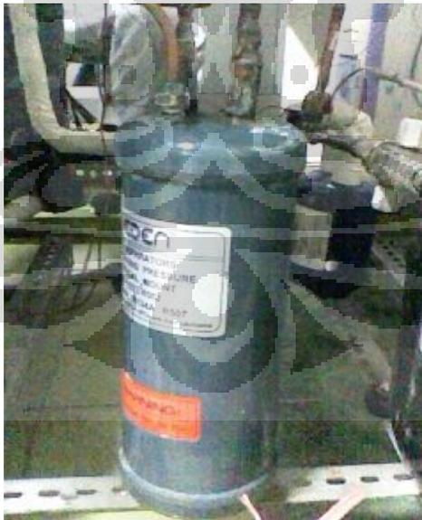
Gambar III-11 oil separator
