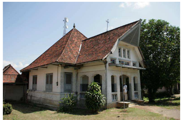
Figure 15. The Former House of Lay A Bah which has an Indische Style (Documentation of Research Team, 2012)
