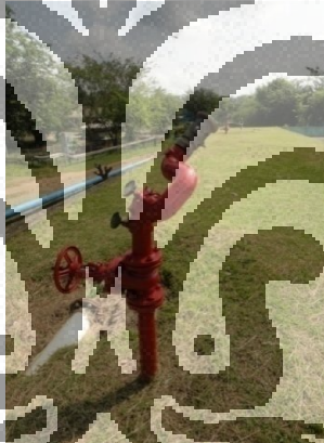
Gambar 6.9 Fixed Monitor
