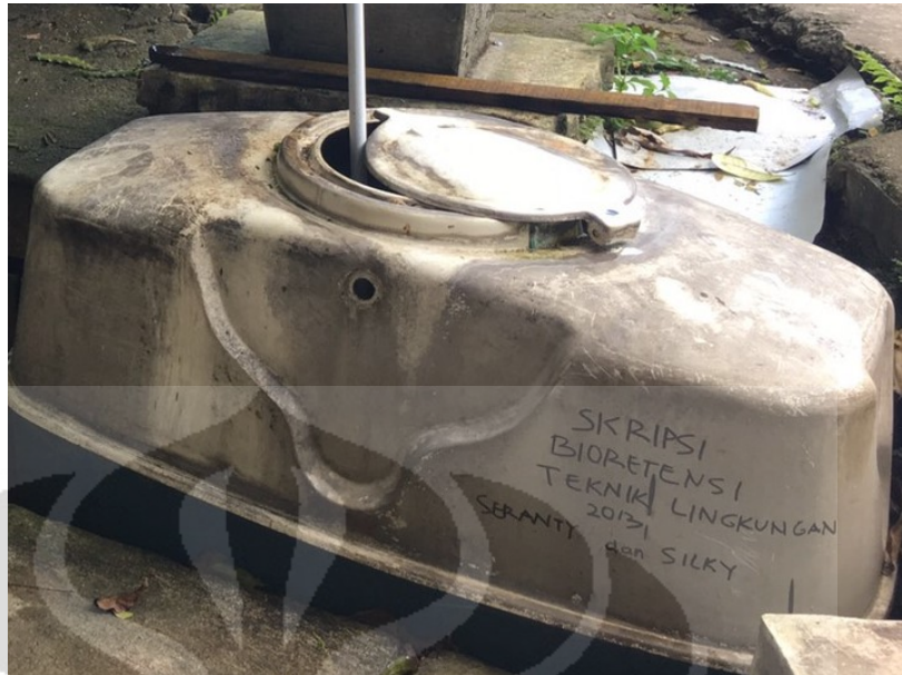
Reservoir Penampung Limpasan Air Hujan
