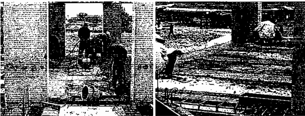
Gambar 5.16. Topping Concrete
