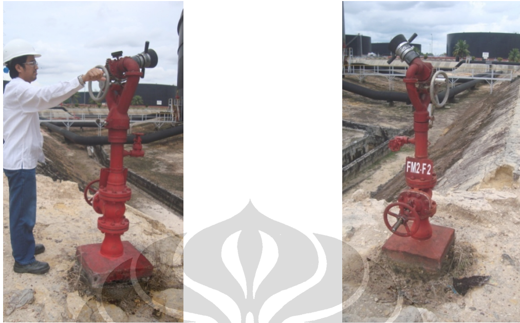
Gambar 9. Fire Monitor
