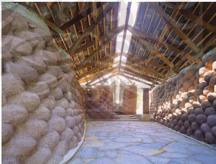
Gambar 14: Dinding dan lantai Yancey Chapel Sumber: Rural Studio
