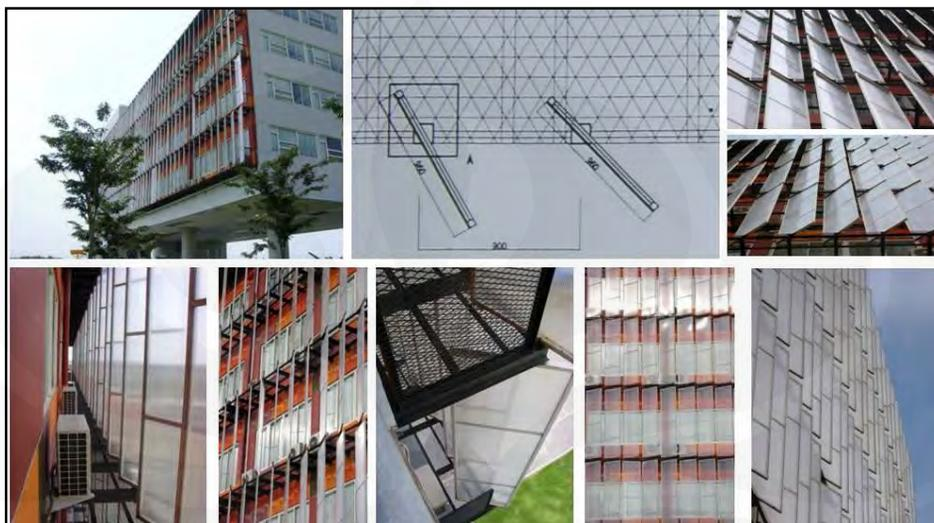
Gambar 4.31 Detail sirip polycarbonate UC
