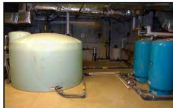
Gambar 3.17 Basement tank & filters Sidwell
