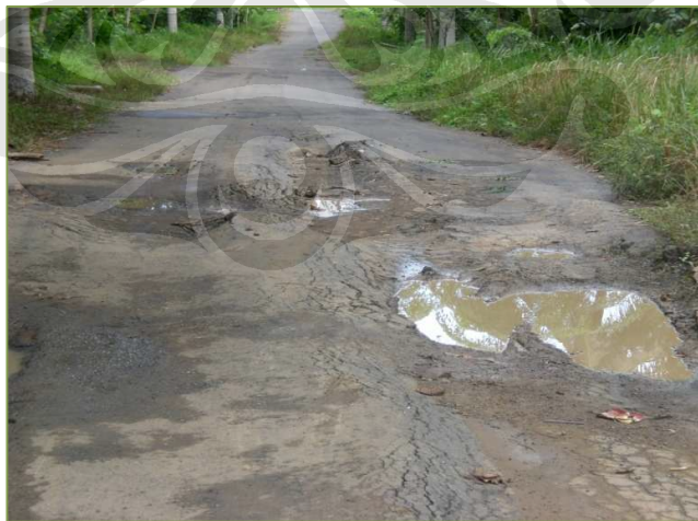
Gambar 3.9 Jalan Aspal 1 km, Youth camp 14
