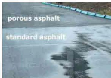
Gambar 2.15 *Porous asphalt* (sumber: [www.porouspavement.com](http://www.porouspavement.com))
