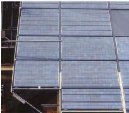
Gambar.68 Panel *monocrystalline silicon*.
