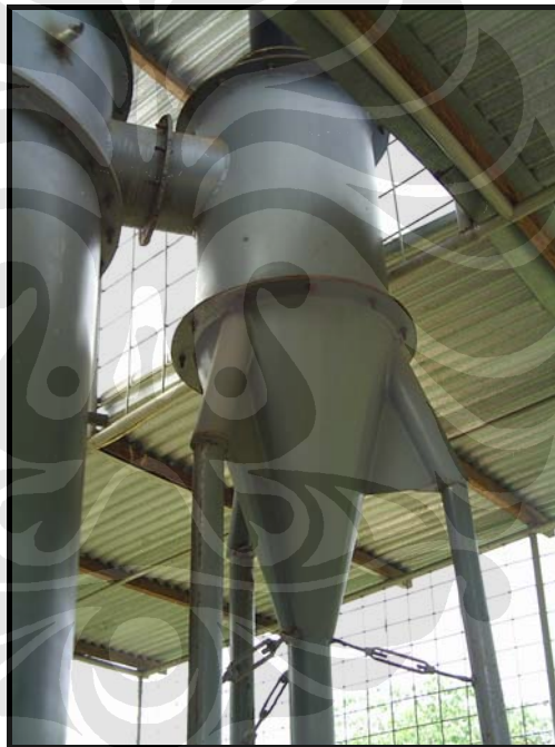
Gambar 2.11. Cyclone separator fluidized bed incinerator UI
