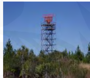
Gambar 2. Airport Surveillance Radar (sumber: http://en.wikipedia.org/wiki/Airport_surveillance_radar , 12 Juni 2008)
