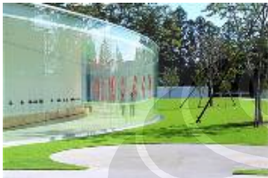
Gbr. 34 : Fasade Bangunan Museum of Contemporary Art Kanazawa
