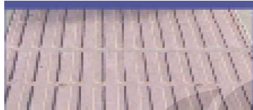
Gambar 2-15 directional surface . (sumber: www.accessforblind.org/dw_presentations.html )
