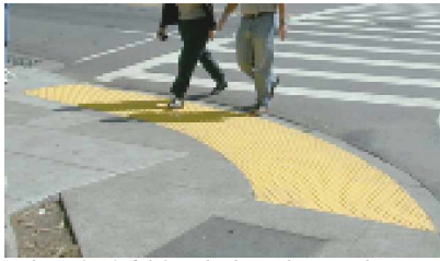
Gambar 2- 26 blended curb (sumber: www.access-board.gov/research/DWSynthesis/DW-synthesis.pdf )
