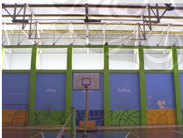
Gambar 4.1.13 Dinding Gymnasium UI
