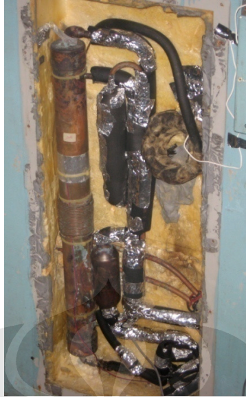
Gambar 4.3 Shell and tube cascade heat exchanger
