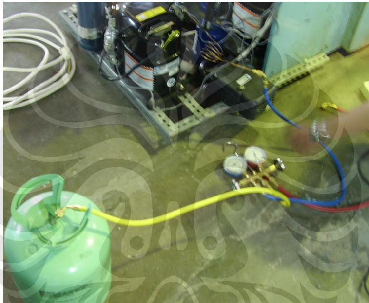
Gambar 4.17 Proses charging refrigeran
