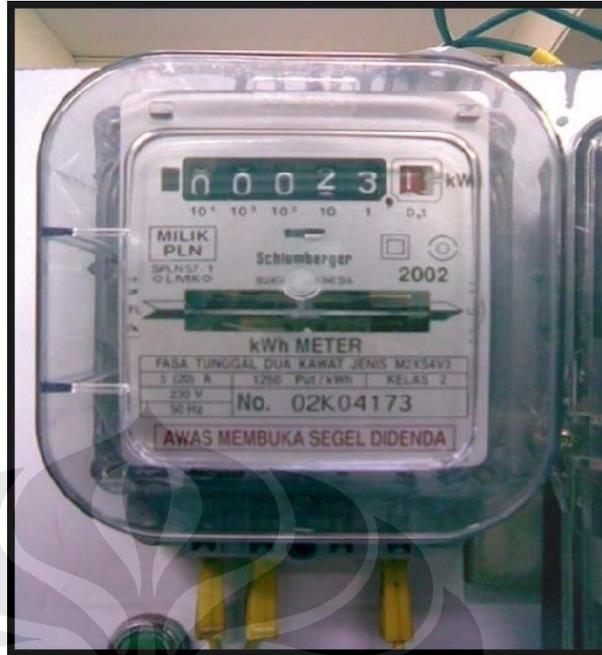
**Gambar 3.2** KWh-meter satu fasa merk Schlumberger
