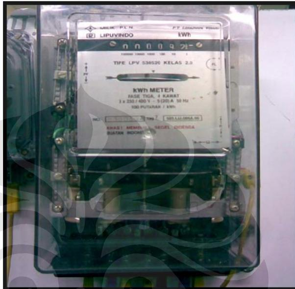
**Gambar 3.4** KWh-meter tiga fasa
