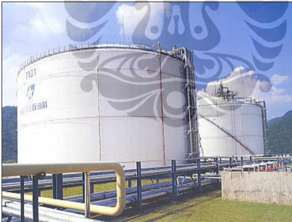
Gambar 2.11a Tangki- tangki penimbunan LPG di fasilitas terminal LPG
