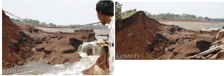
Figure 3 Collapse of Gintung Situ
