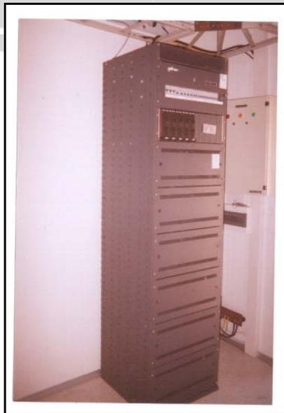
Gambar 2.3 *Rectifier Power One PPS16.48* [15]
