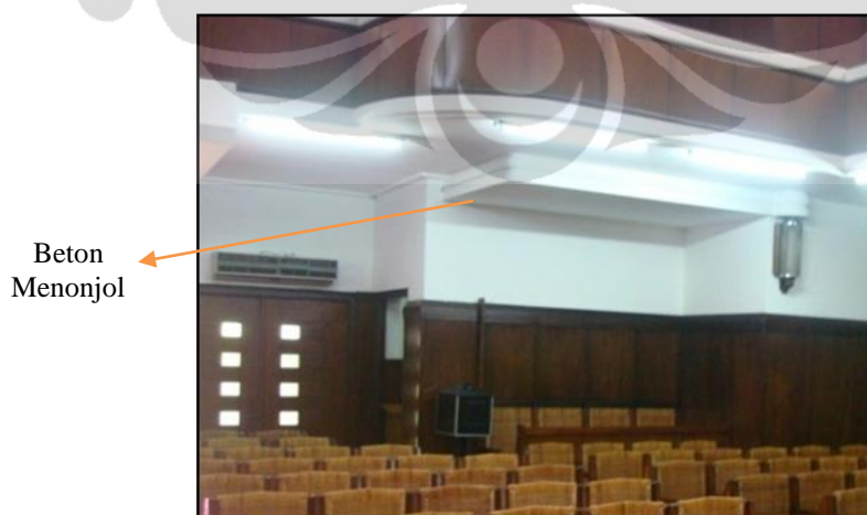
Foto 2.47 Beton Menonjol (Dok. Achmad Ghazali, 2010)
