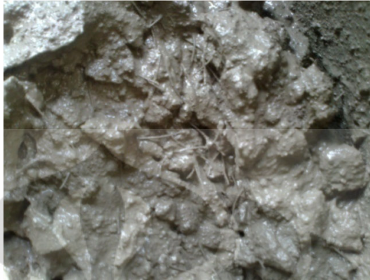
Gambar 4. 9 Beton Segar Hasil Mixing
