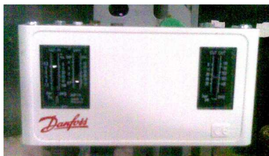
Gambar 3. 9 Hi-lo pressure control merk Danfoss.
