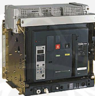
Gambar.3.3. Air Circuit Breaker (ACB)
