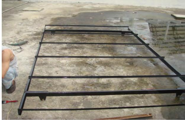
Gambar 3.3 Bracket solar cell
