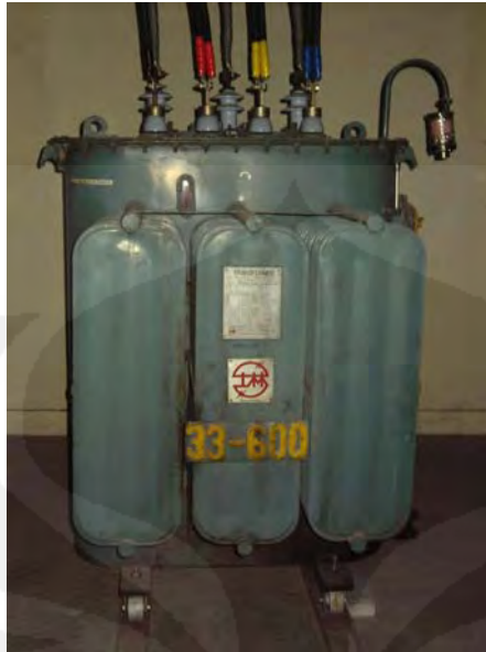
Gambar 2.7. Tranformator Distribusi
