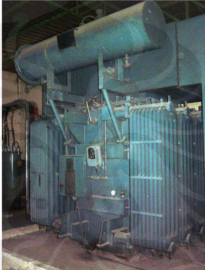
Gambar 2.6. Tranformator Daya
